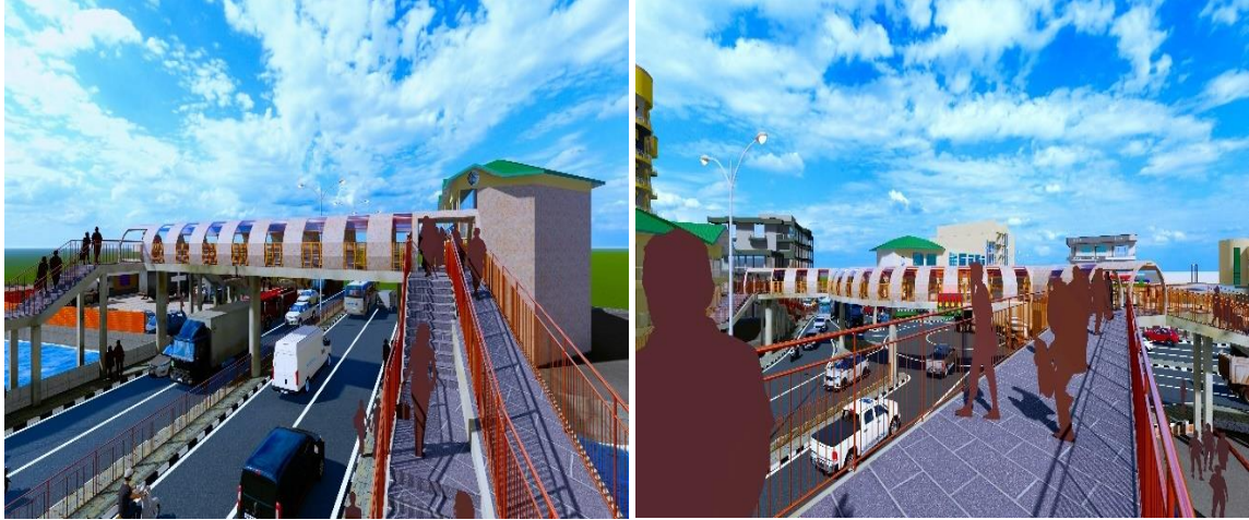
Figure 18: Ramp and Stair of proposed pedestrian bridge.
