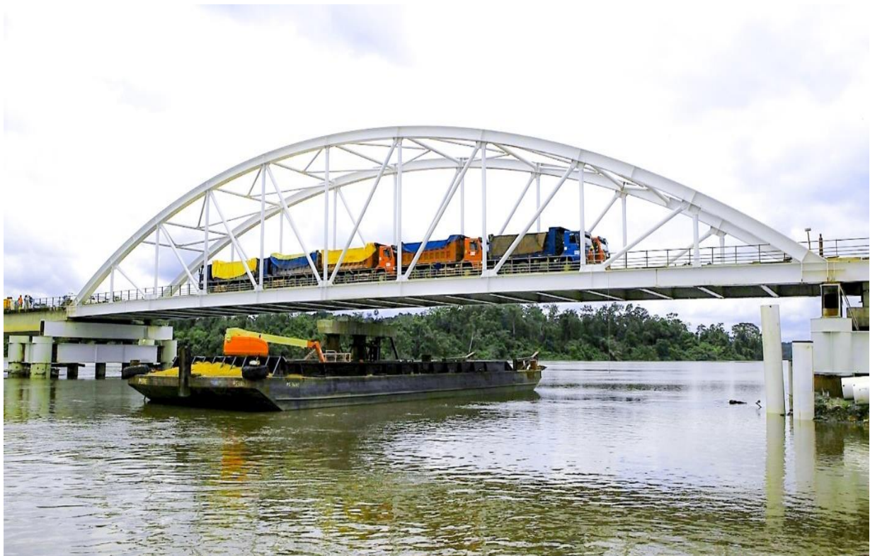
Figure 3.1: KANGO bridge to be renovated
