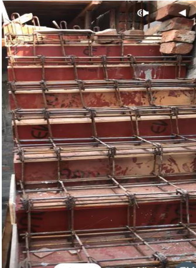
Figure 4 . 12 : Stairs structural reinforcement
