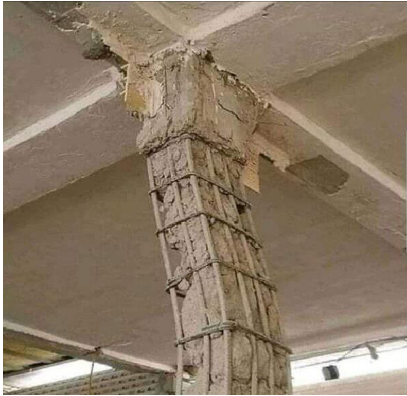
Figure 2.4: Buckling
