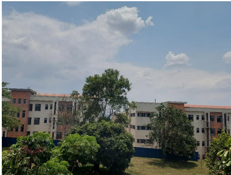
ULK hostels green building which is under construction.
